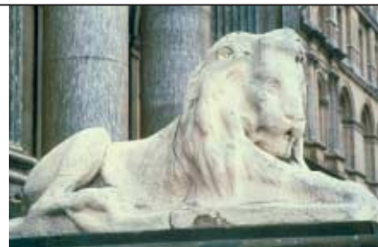
Figure 6 ▶ This stone lion sits outside Leeds Town Hall in England. It was damaged by acid precipitation, which fell regularly in Europe and North America for more than 50 years.
